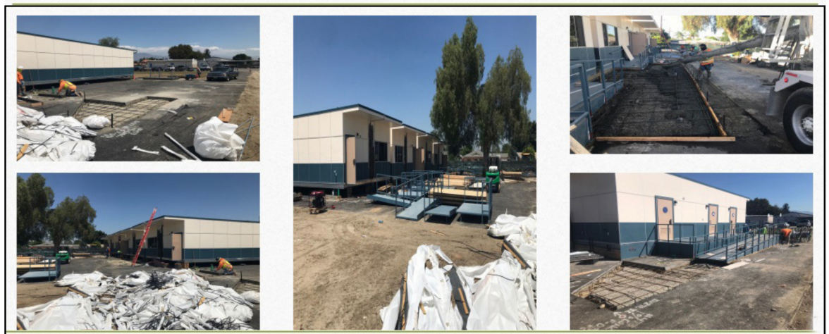
Installation of Portable Classrooms and Restrooms
