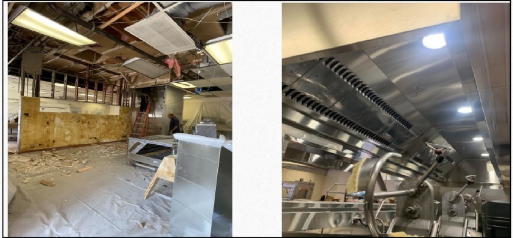
Central Kitchen Modifications
