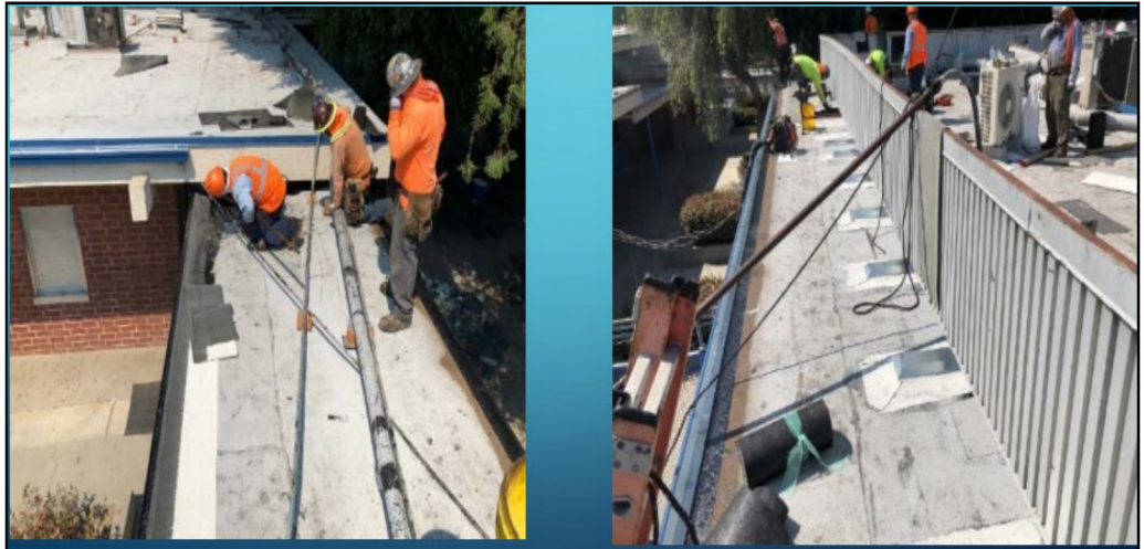
Roofing Replacement and Repair
