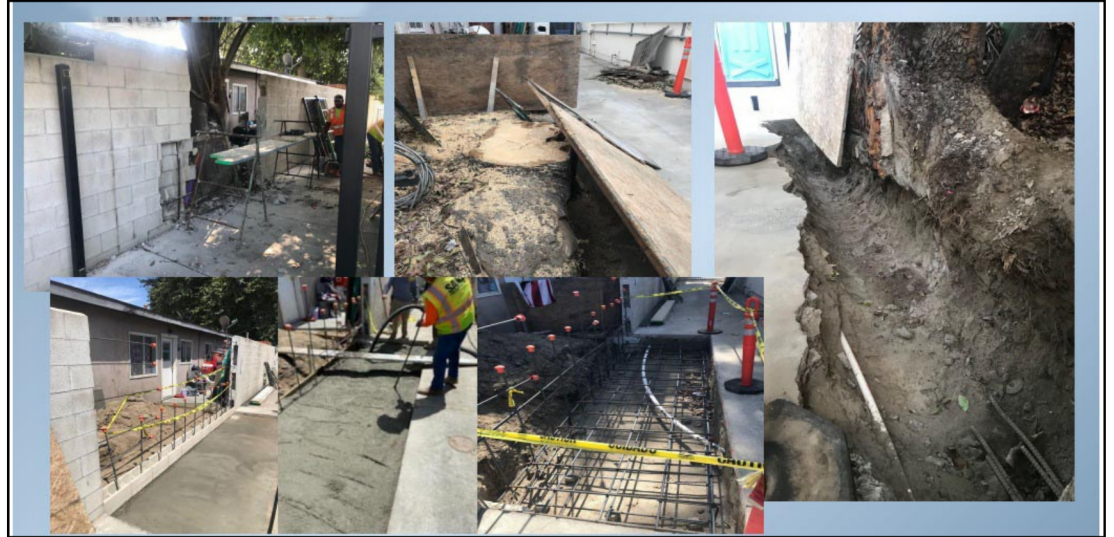
Tree Removal and Block Wall Repair
